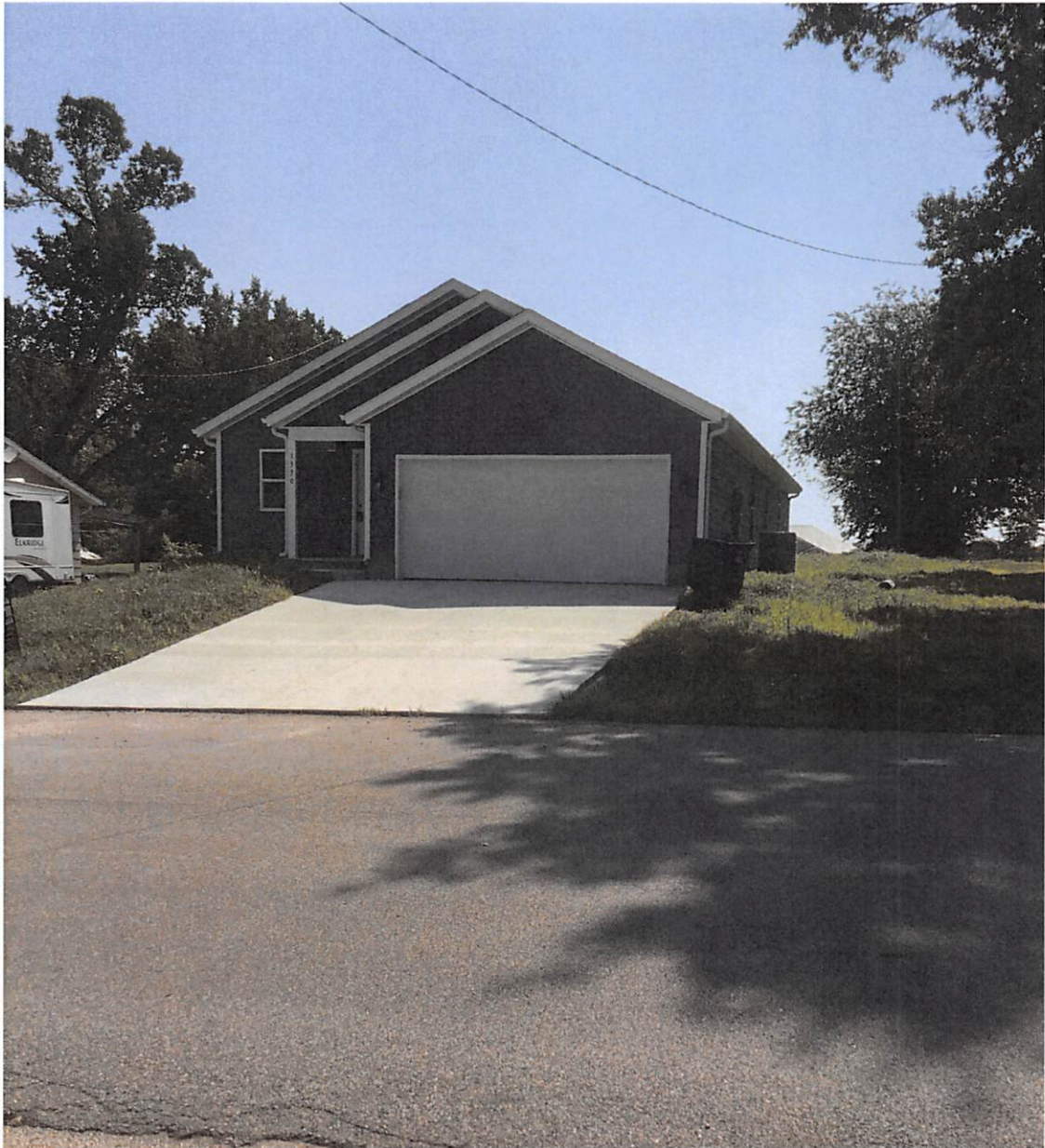
1330 Glenwood (South side)
