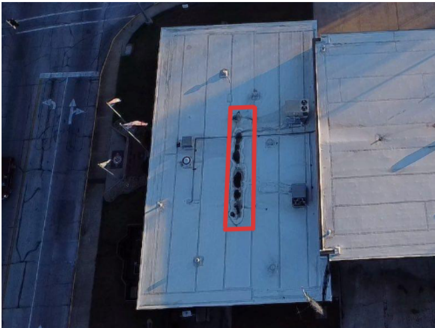
Area of pond filler application.
